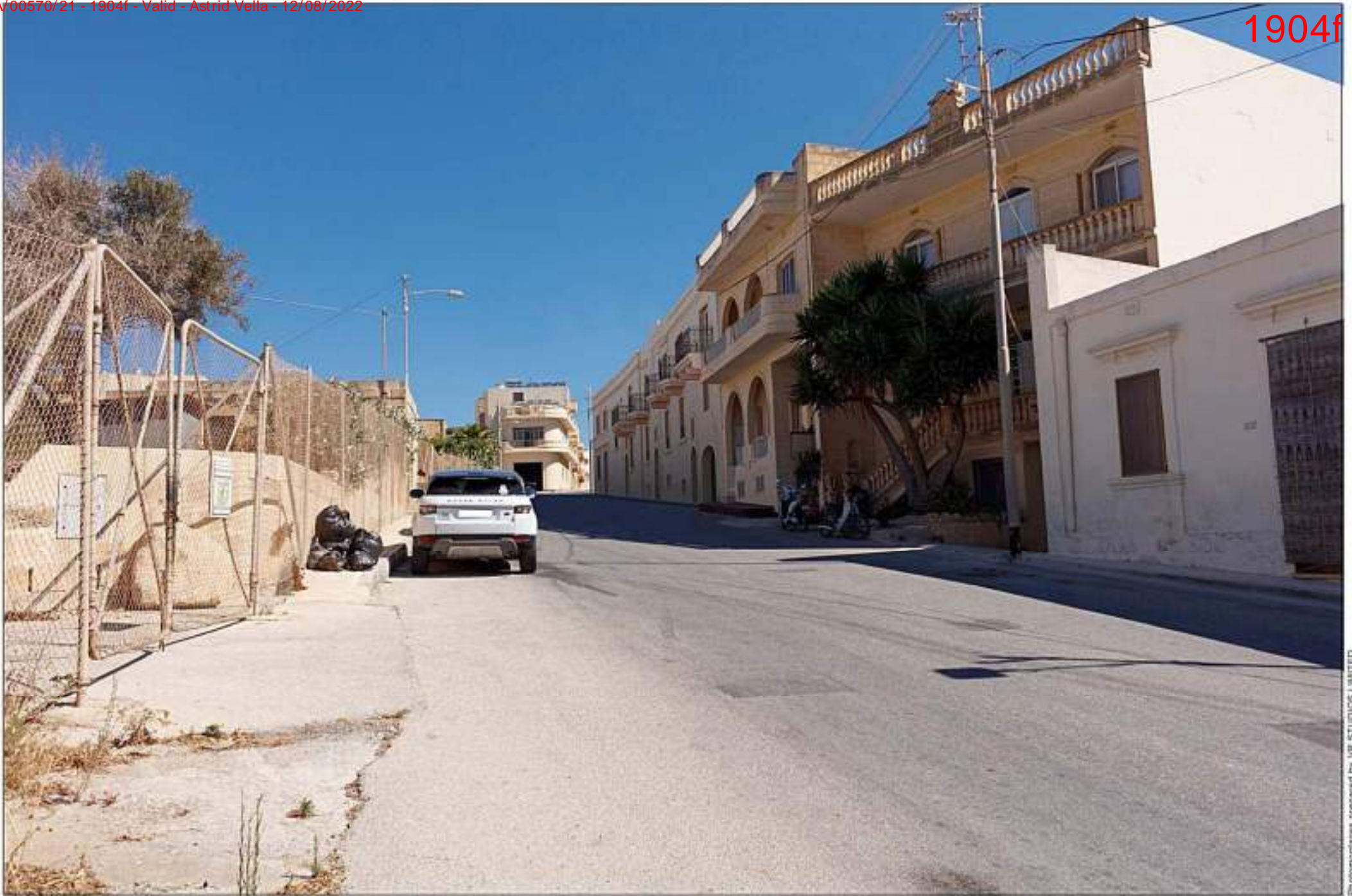
VIEWPOINT REFERENCE 02 YR 0 - 10 Distance to proposed development: 38m Camera height: 1.5m Date & time of photograph: 14-Jun-21; 1020 VFOV: 46.4 deg HFOV: 65.5 deg Date: 31-May-22
